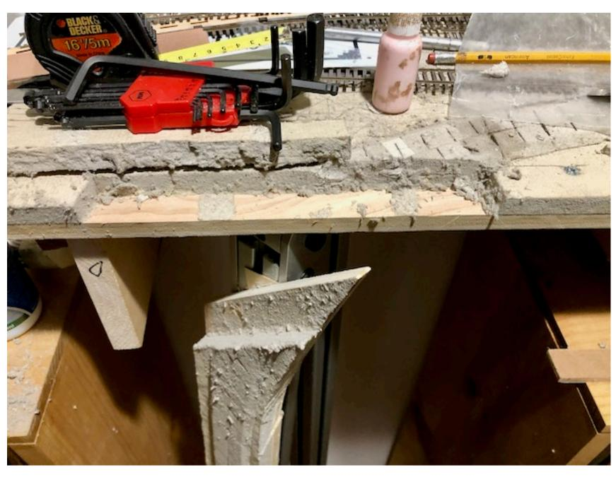
Also I glued some pieces of 1/32 plywood to get a piece of 1/2 homasote to the correct height. The glue is drying today, tomorrow I can cut that piece into strips and test-fit into the notches. I'm sure I'll need to do more filing/sanding to get rid of the glue residue and get everything back to level. dave
